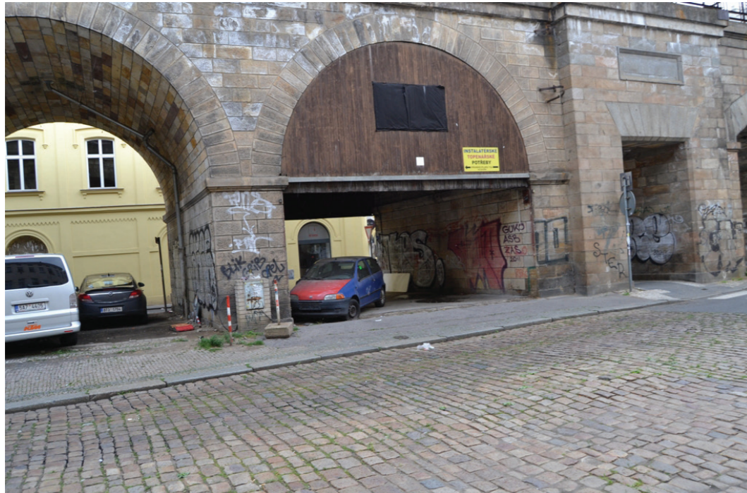
ATMOSPHERE OF THE VIADUCT BEFORE CCEA INTERVENTIONS
